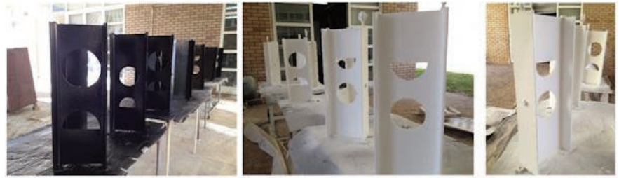
Figure 4. Application of the primer and intumescent coating to the profiles.
